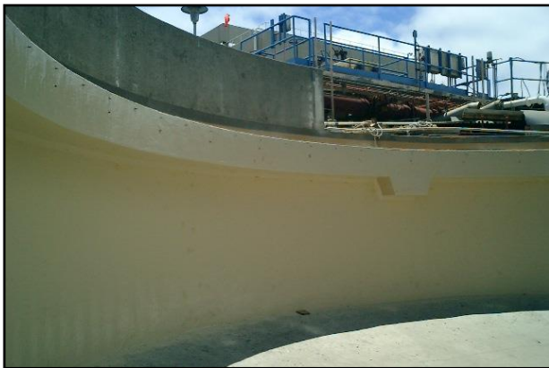
View of completed walls protected with SewerGard 210G
